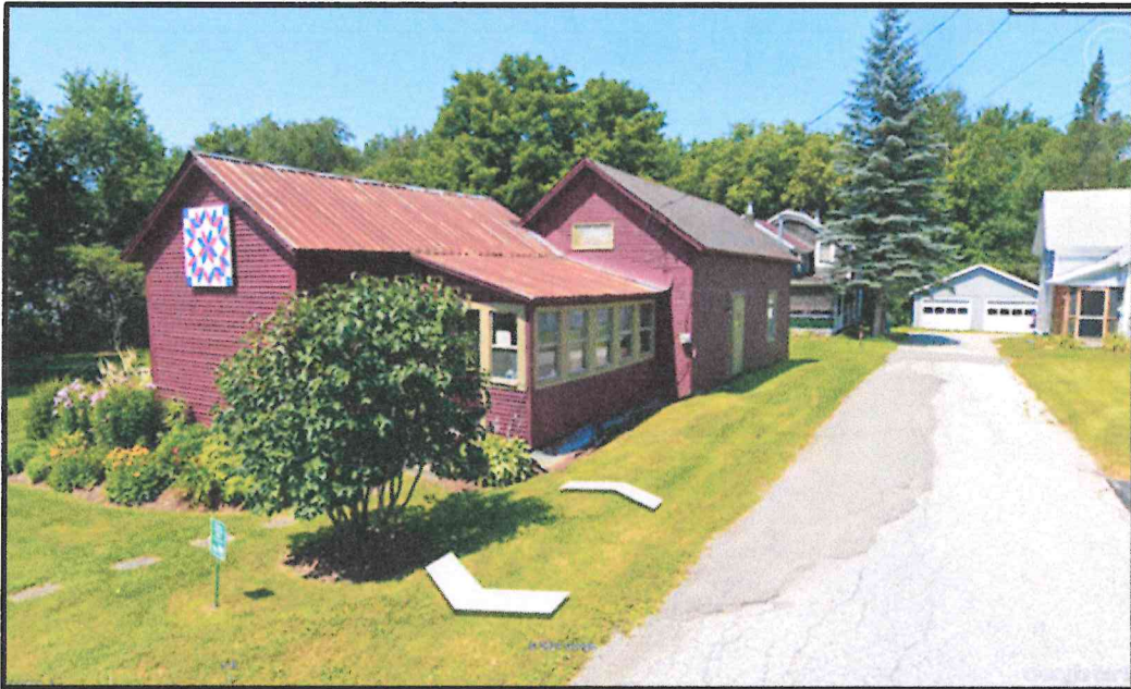
Existing building on Deuso Road
