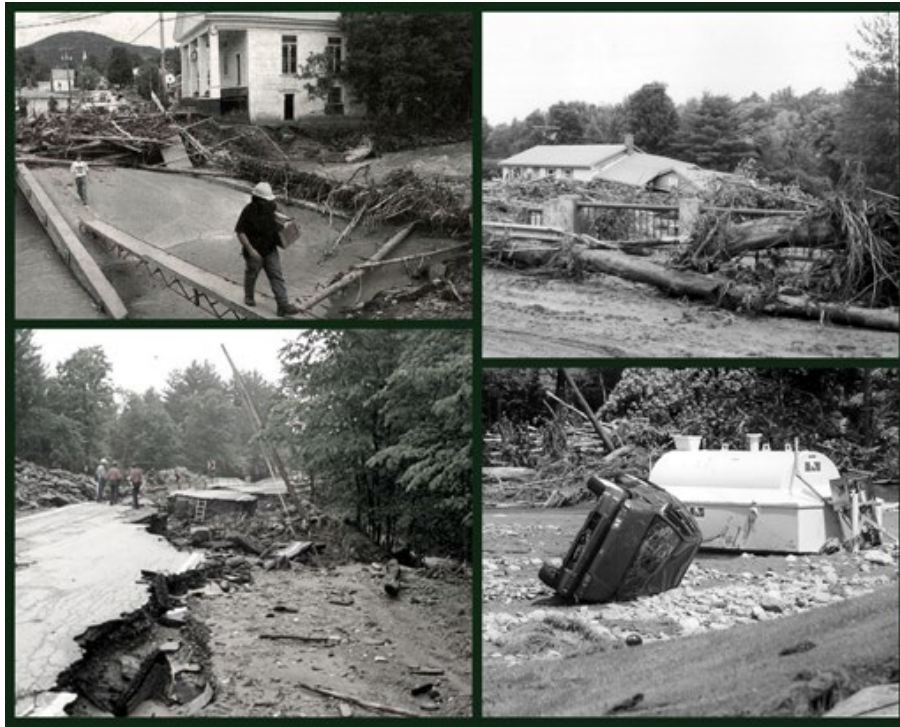
Montgomery Flood July 15, 1997
