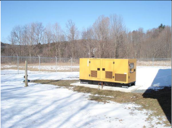
Back of Water Plant
